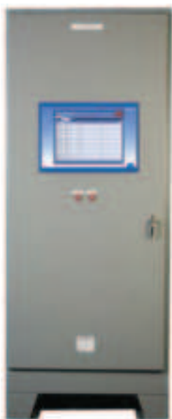
Figure 1.1 Touch 1500 mounted in the NGC-40 panel
