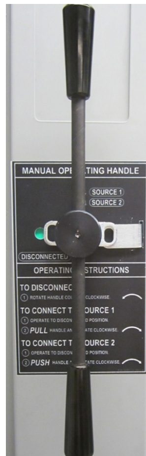
Figure 3. DISCONNECTED (from SOURCE 1 or SOURCE 2) position indicator
