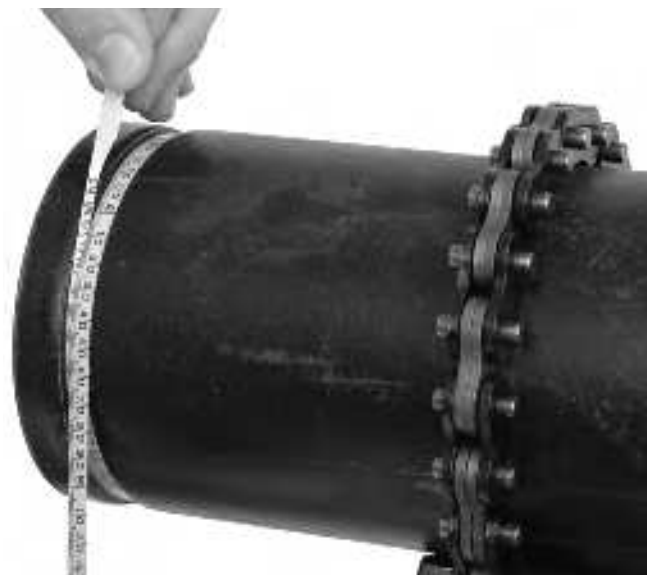
Figure 21 – Checking Groove Diameter with a Diameter Tape
