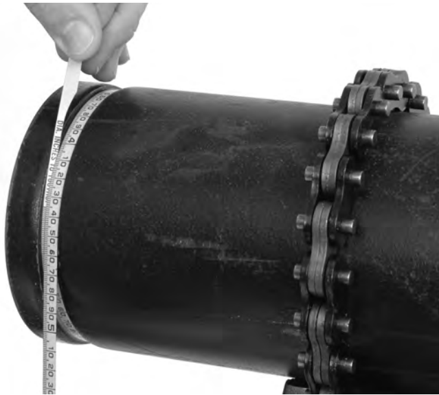
Figure 21 – Checking Groove Diameter with a Diameter Tape
