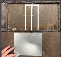
5 Insert the SpeedFlash® Shield fully as shown.
