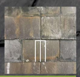
4 The SpeedFlash® Shield is used to protect a specific area of the course below when cutting the top slate(s).
