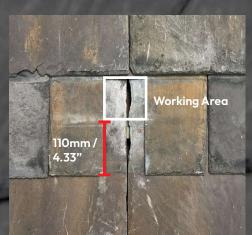
7 Using the angle grinder, cut out the 'working area' on the slate i.e. the area from the 110mm / 4.33" horizontal line and the 190mm/7.5" horizontal line.
