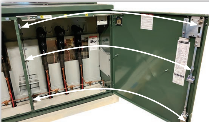
FIGURE 7. Two-step controlled opening of doors.
