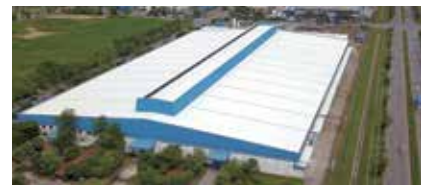
Fujitsu General (Thailand) Co., Ltd. (Thailand) FACTORY-2
