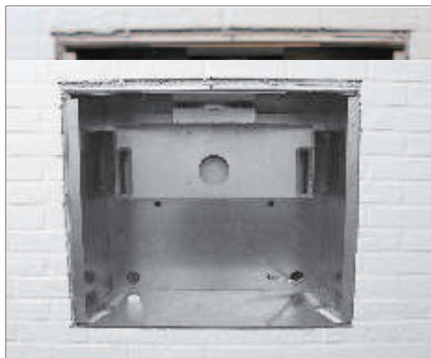
Zero Clearance Box and coaxial flue adapter
