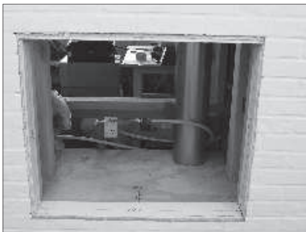
False Fireplace enclosure
