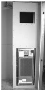
Figure 15. Install chassis centered
