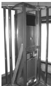
Figure 8. Mock-up of stud placement
