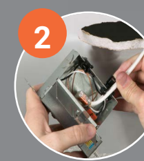
Connect wiring to junction box.
