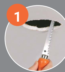
Cut hole in ceiling.
