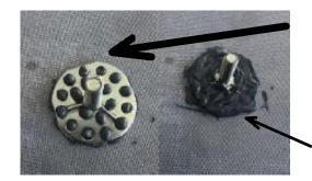
Lastly, take the Sink Clip and push firmly down onto the cleaned Countertop Underside. Press firmly and wiggle around some to assure all gaps are covered. You will notice some epoxy will seep through the holes, take your mixing stick and add extra epoxy to the top to cover the Sink Clip for better bond result.
