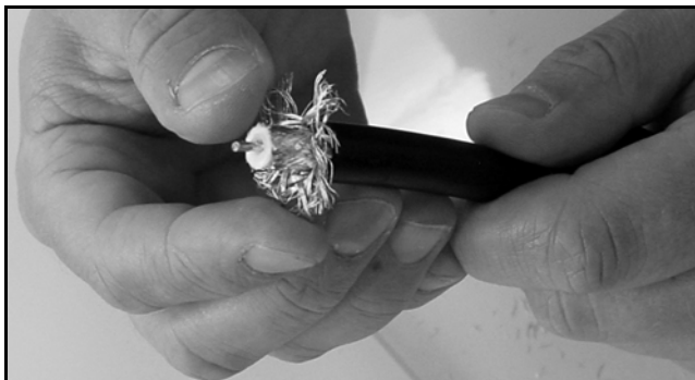
Figure 92: Flaring the Braid
