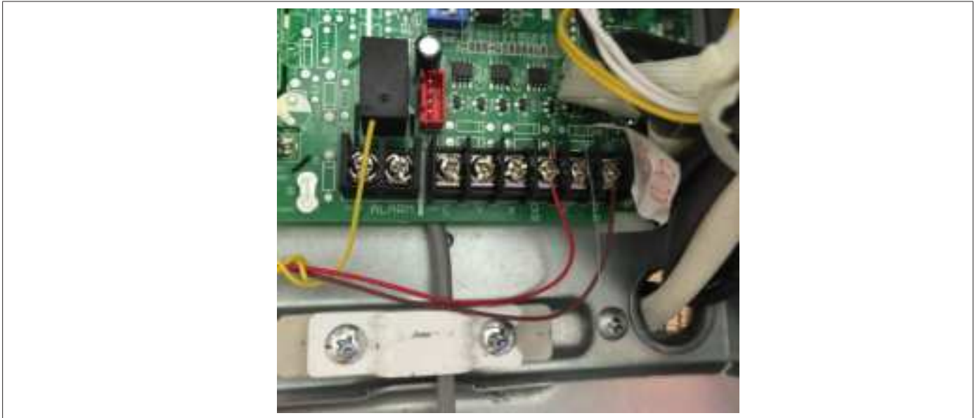
Figure 16. Alarm Device Connection Points (Typical)
