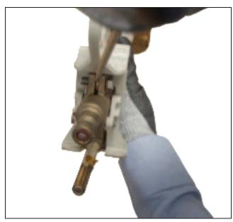
Figure 6. An SM-20 Fuse Unit upper end-fittling showng a screwdriver prying the clamp and spacer washer slightly apart, after loosening the clamp screw, as part of the fuse-replacement procedure.
