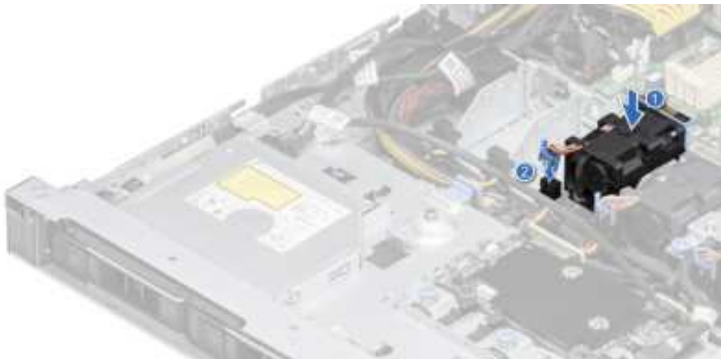
Figure 24. Installing a cooling fan
