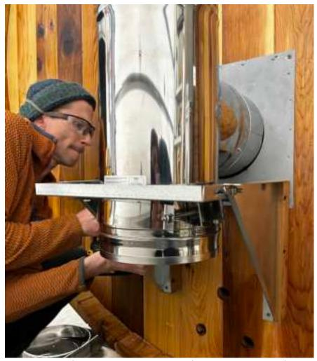
(make sure to install the support brace in a way that doesn't obstruct the bottom cap from being opened)
