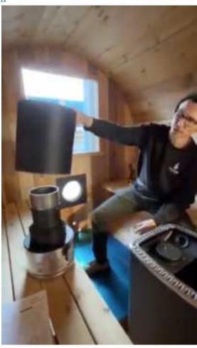
Next, move the stove back towards the wall until the insulated pipe section passes into the port. When the stove is in position, the black finishing cover will be snug against the stove on one end, and snug against the wall on the other end.
