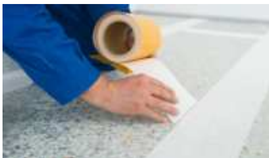
Fig. 9: Tape up short butt ends as well but do not allow the tape to overlap.
