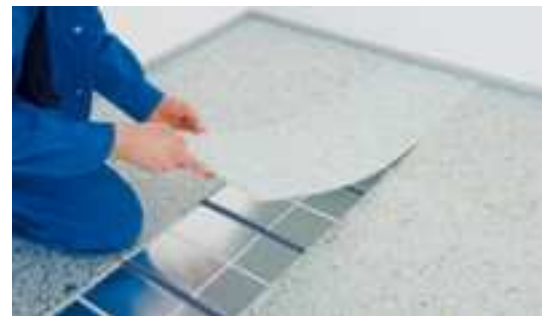
Fig. 4: Panels cut length-wise should be laid in the penultimate rows and care should be taken to keep the staggered pattern.
