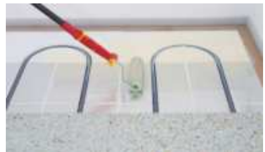
Fig. 6: Always use an adhesive to fix Strongboard to the heat panels.
