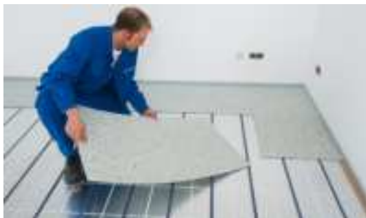
Fig. 3: Continue laying the Strongboard panels in a staggered pattern. Always use whole panels along the edges.
