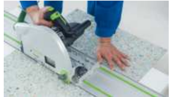
Fig. 2: Cut Strongboard with circular saw (universal blade). Use off-cuts at beginning of next row.
