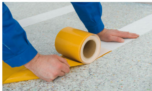
Fig. 8: Tape up all butt joints with 140 mm joining tape.
