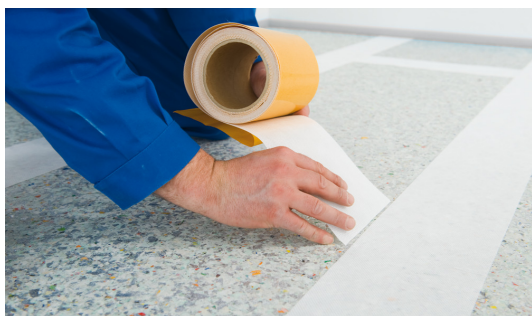
Fig. 9: Tape up short butt ends as well but do not allow the tape to overlap.
