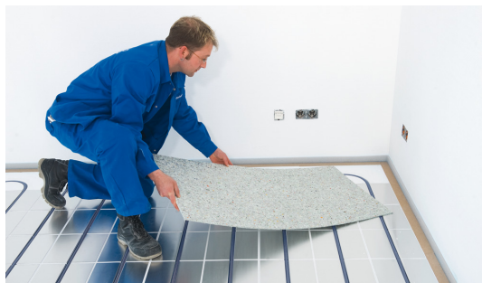
Fig. 1: Before applying adhesive, lay Strongboard in staggered pattern (see 3) onto the evenly laid heat panels.
