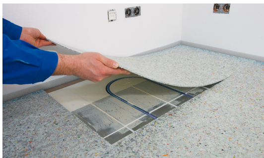
Fig. 7: Allow the adhesive (e.g. Ecofix by Mapei) to evaporate for 10 mins before continuing to lay the panels.
