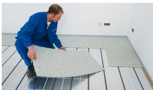
Fig. 3: Continue laying the Strongboard panels in a staggered pattern. Always use whole panels along the edges.
