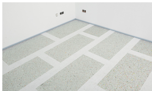
Fig. 10: Protect the finished floor from dirt and from pedestrian traffic to avoid damage with e.g. insulation panels.
