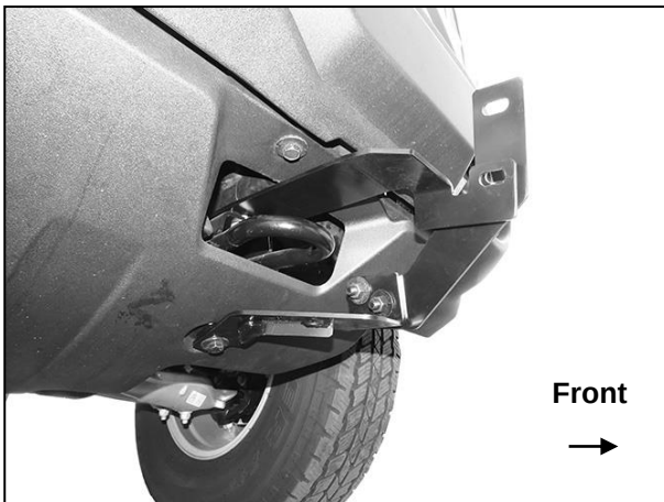
(Fig 11) Driver/left side Brackets installed
