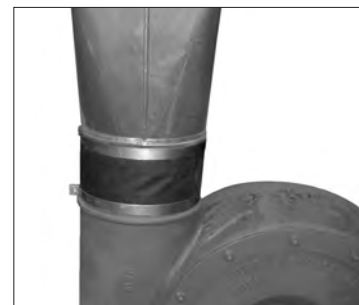
Installed Duct Connector
