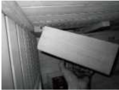
FIG-16 Installing the Radio Wood Housing
