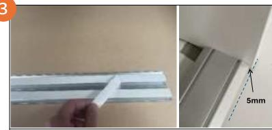
Position the bottom track ensuring it is placed **5mm** in from the front of the wardrobe before securing. If a packer has been provided, this needs to be screwed/glued to the hard surface under the bottom track first. when ready to secure, peel off the backing of the double-sided tape and mount in place.
