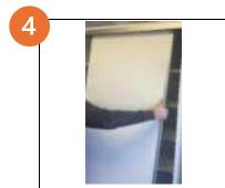
Slip the top of door into rear channel then set bottom onto the rear floor track by pushing up the bottom wheels to help slot in place. Repeat for second door using the front channel.
