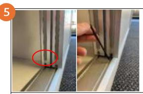
Pull up the bump stop enough to reveal the adjusting hole. Use a 4mm allen key to adjust wheels. (Clockwise to raise or Anti-clockwise to lower). This adjustment helps ensure the doors align properly with the door jambs.
