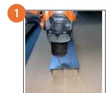
Use a 5mm drill bit to pre-drill mounting holes for the top track where necessary.
