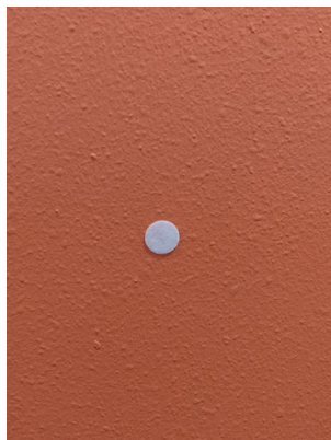
Stick Velcro on wall at equipment location
