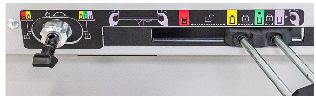
Interlock Operator in the Locked Position; Withdraw Lever in the Disconnected Position.
