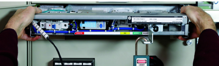
Withdraw lever in Released position (and locked out).
