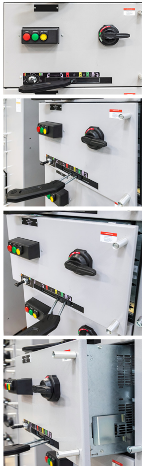
Figure 36 - Various Positions of Withdrawal Units with SecureConnect
