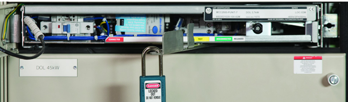
Withdraw lever in Test position (and locked out).
