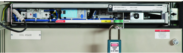
Withdraw lever in Disconnected position (and locked out).
