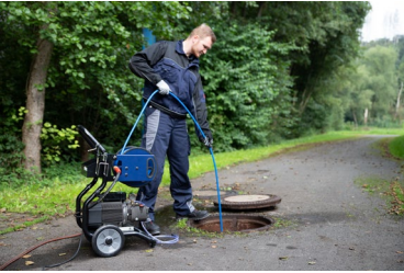
Fig. 36: Washing a pipe using the hose
