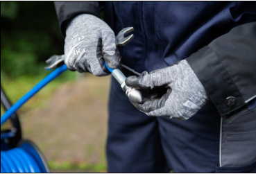
Fig. 32: Screwing on the pipe washing nozzle
