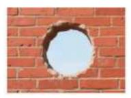
2.Insert the product into the open hole, mark the wall with two screw holes of the product as a reference, and drill holes on the two marks. The outer diameter of the hole is 3mm and the depth is 40mm
