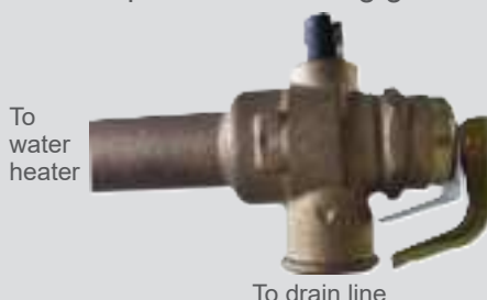
How to operate the easing gear
