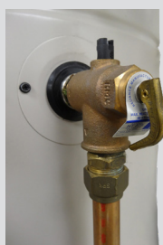
TPR position - top of cylinder
