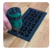
Screw in the registers from the pre-drill holes. If your vent does not have pre-drill holes, make sure to add before installation
