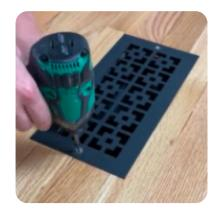
Screw in the registers from the pre-drill holes. If your vent does not have pre-drill holes, make sure to add before installation
