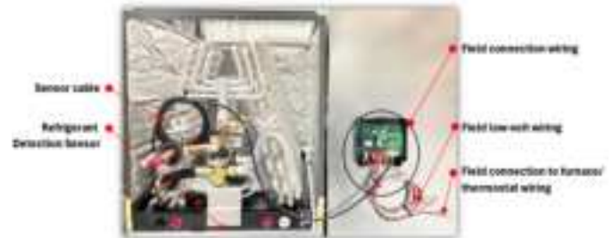
Fig 12.3 A - Mitigation Control System
