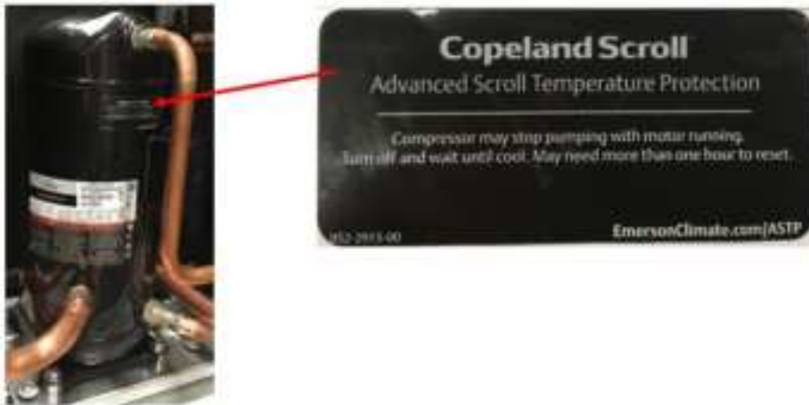
Figure 13: Advanced Scroll Temperature Protection (ASTP)
