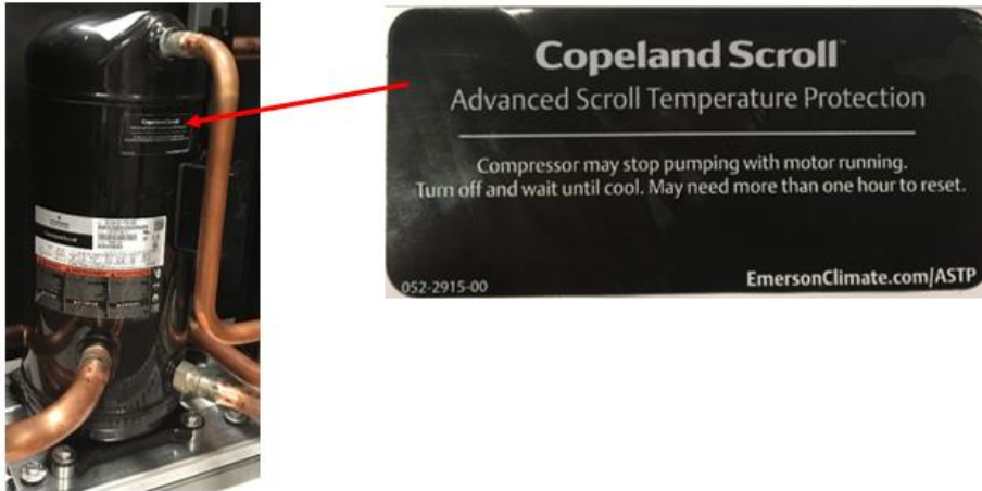
Figure 13: Advanced Scroll Temperature Protection (ASTP)
