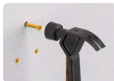
Install the wall anchors
