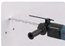
Drill holes on the wall
