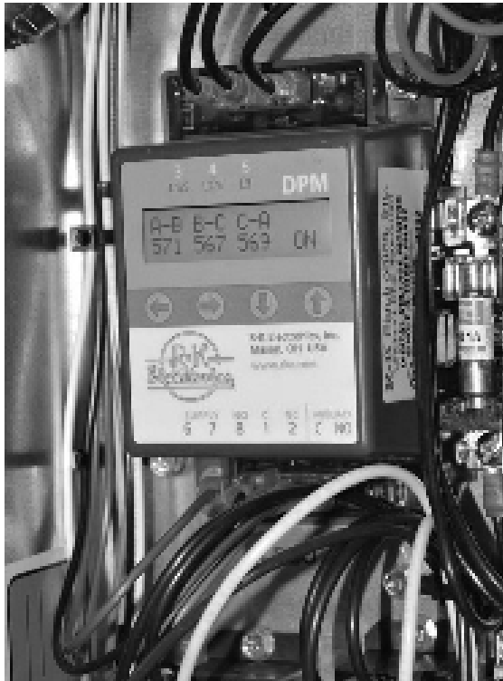
Figure 78 – Digital Phase Monitor
