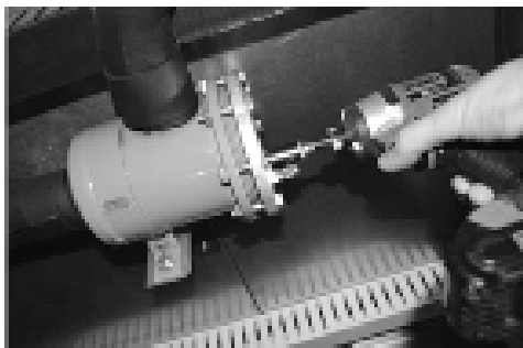
Figure 52 — Remove Pleated Filter
