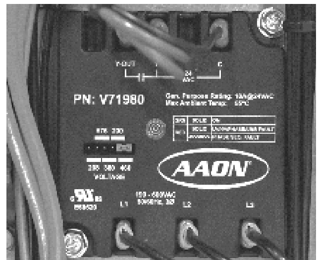
Figure 79 – Phase and Brownout Protection Module
