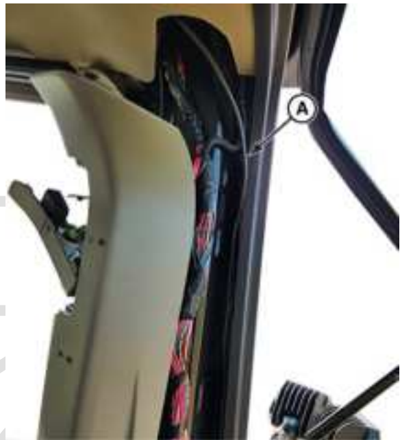
Antenna Cable Routing
