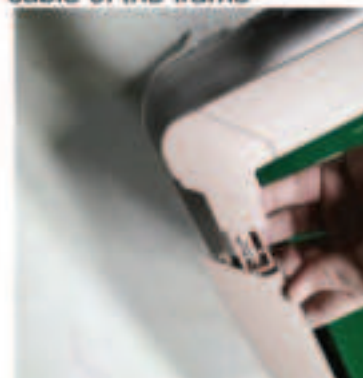
Step 9: Install the edge cover
