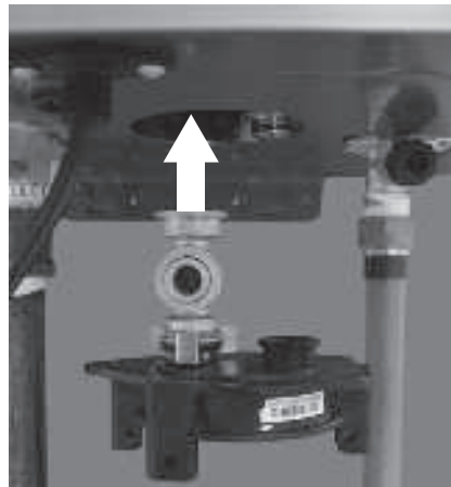
Figure 251 - Orient cartridge manifold and outlet tee
