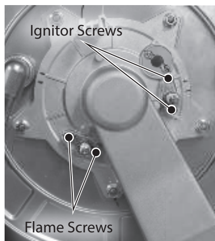
Figure 116 - Remove ignitor rod and flame sensor screws
