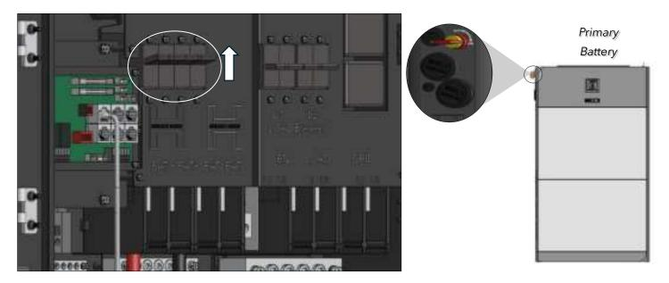
2. Turn ON the Disconnect on the eWay. For paralleled battery systems, **only** turn on the Primary Battery
