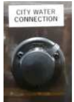
City Water Fill w/Connection Label
