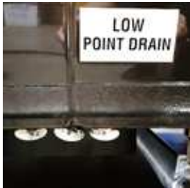
Low Point Drain Example
