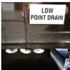
Low Point Drain Example
