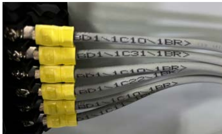
Control Wire Marking
