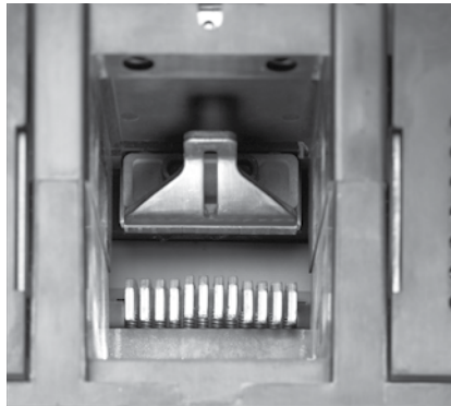
Magnum PXR Breaker Contacts (Arc Chutes Removed)
