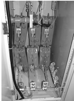
Grounding Balls and Covers
