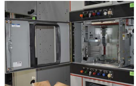
Bellows and Two-Point Door Latch
