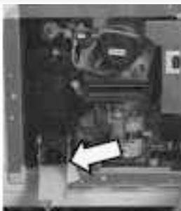
Draining the Aqua Go Water Heater
