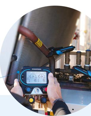
This tool allows the user to commission a heat pump, check the refrigerant circuit tightness or fill gas and check differential pressure and subcooling / superheating temperatures simultaneously.
