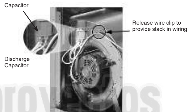
Figure 3: Discharge Capacitor and Release Wire Clip
