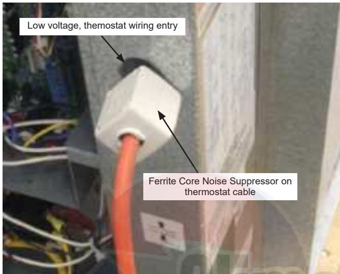
Figure 39: Ferrite Core Noise Suppressor on Thermostat Cord Cable
