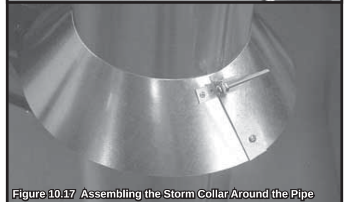
Figure 10.16 Assembling the Storm Collar
