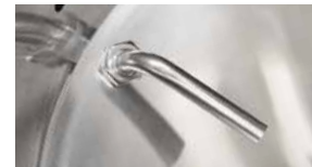
Tail piece installed
