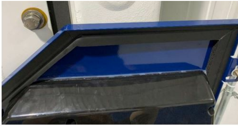
Figure 7b: Caulking of Rain Shield
