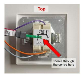
• Step 3: Insert the humidity sensor/LED
