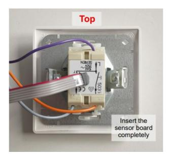
Step 4: Install the control unit and switch in a flush-mounted box – done
