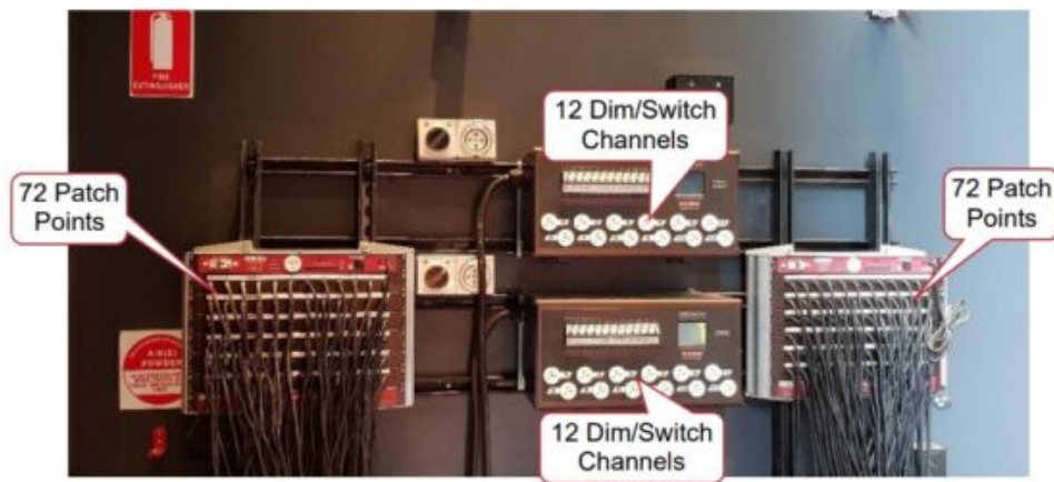
Typical Installation. 144 Patch Points and 24 Dim/Switch channels
